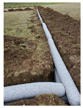
Figure 3 –Tile dewatering trenches were installed 15-52 inches below grade and filled with 12" EzFlow bundles. 4" pipes at the bottom of the trench sloped are at 0.2-0.4%.
