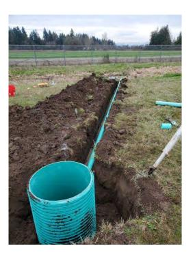
Figure 4 –24" silt traps were installed at the inlet end of each tight line outfall, which discharged toward existing drainage swales on the site. Photo taken facing west toward the west property line (fence) with Hubbard Cuttoff Rd. NE in the background.
